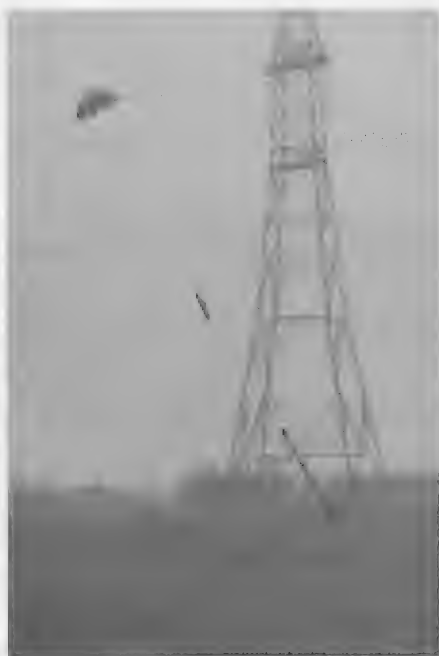
Figure 7-44 Snagged in a pylon.
